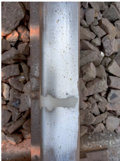
Fig. 7. Rail surface after application of Belzona friction component [photo: S. Grulkowski]
