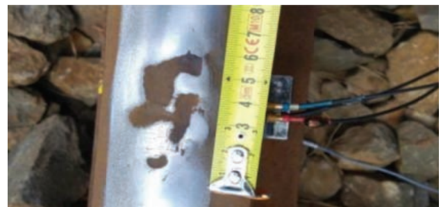
Fig. 3. Example of a "squat" defect [16]
