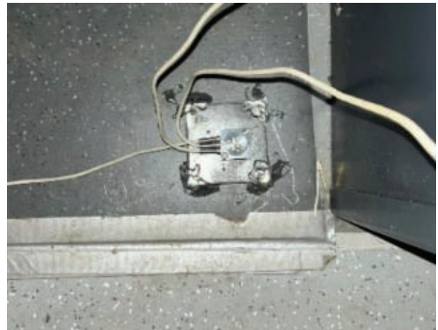
Fig. 10. Measurement point 2 localized on the train floor [photo: A. Łomżyńska]
