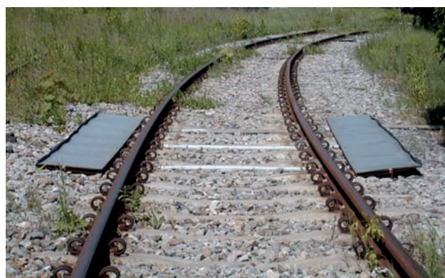
Fig. 12. Measuring curve built in accordance with EN 14363 [12] method no. 1 [photo: A. Chojnacki]
