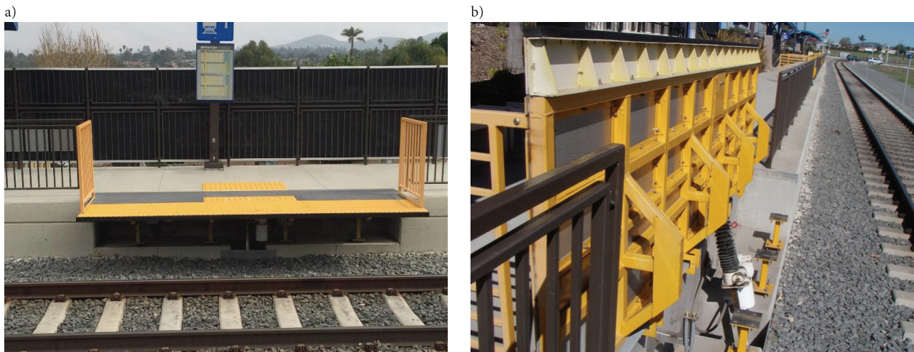
Fig. 12. View of a laid down footbridge (a) [4], laid up footbridge (b) [20]
